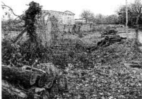
Wood clearing prior to work commencing
