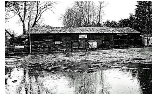
The original scout hut before demolition
