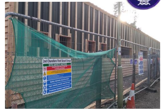
Work progressing well with wooden cladding going on
